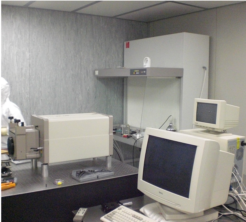
Figure 54: Zygo GPI-XP installed at Luxor clean room.
