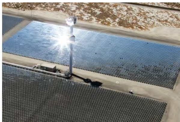
Figure 4-6: grid layout in the Sierra Sun Tower by eSolar ( www.solaripedia.com )
