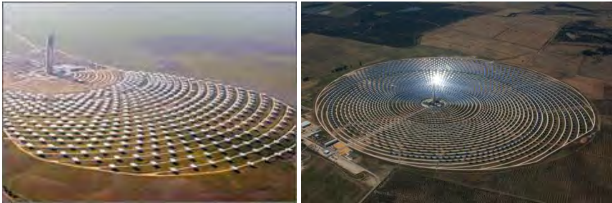
Figure 4-5: left, PS10 north field ( www.nrel.com ); right, Gemasolar surrounding field ( www.torresolenergy.com )
