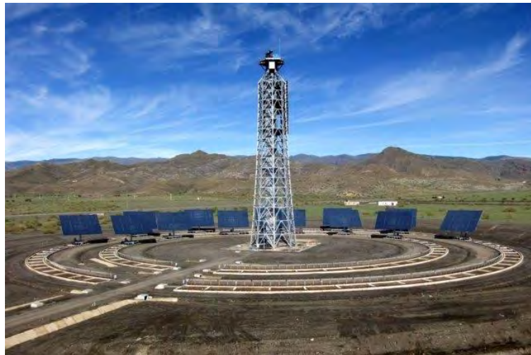
Figure 4-9 Variable-geometry solar field at CTAER (Centro Tecnológico Andaluz de Energías Renovables) ( www.ctaer.com )
