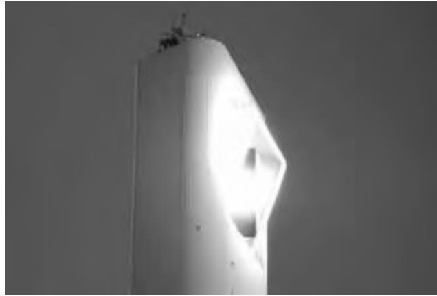
Figure 4-16: spillage loss at PS10 receiver
