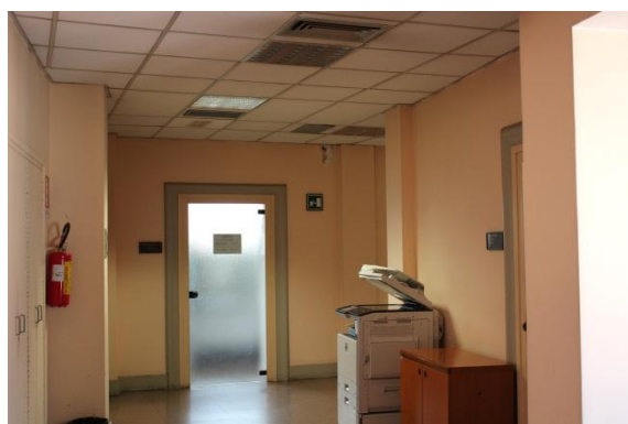
Fig. 3.2-22: 3P: corridoio, ala sud.
