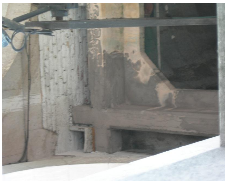
Fig. 6.2.4-04: Trave a T e soletta in c.a..
