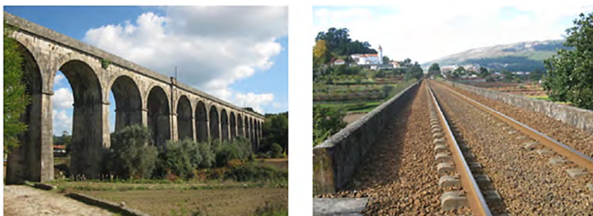
Figure 4.1: Durrães viaduct and binary detail
