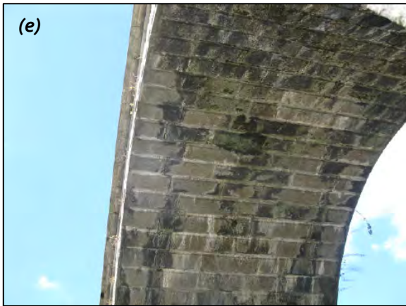
(e)Cracks in right and left side of the arch depth in arch 2
