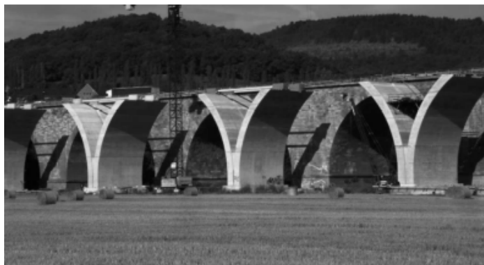
Figure 2.16: New Saale Bridge South Jena (Proske, et al., 2009)
