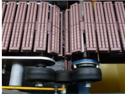
(b) Idler pulleys of an elevator.
