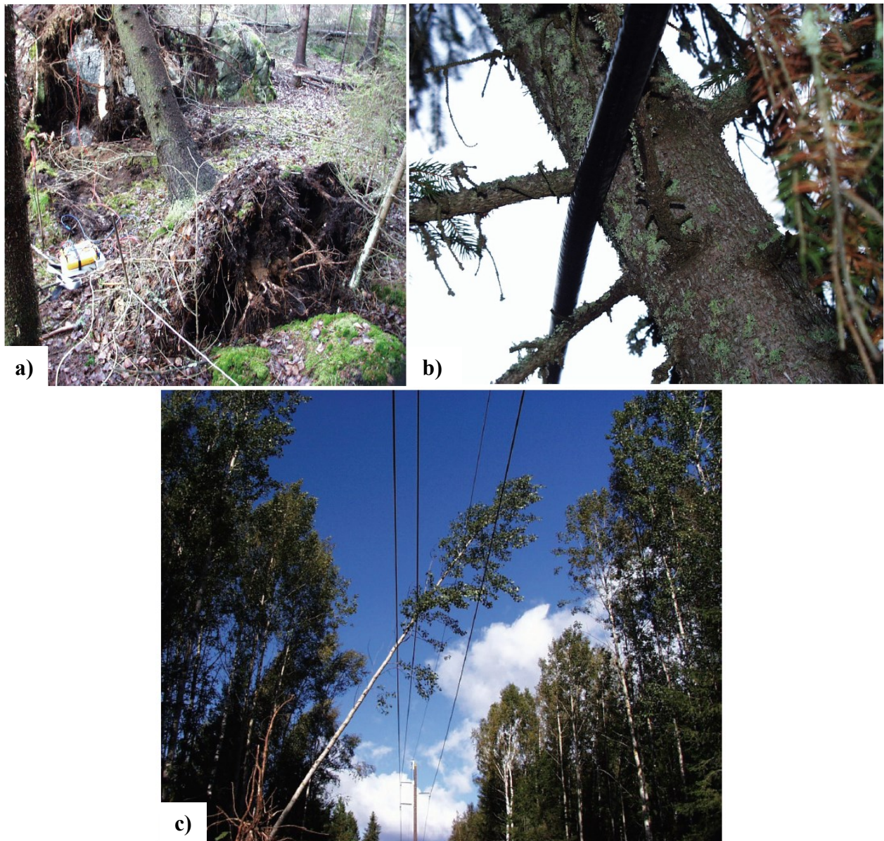
Figure 2.11 Steps of test arrangement: a) the roots of a tree felled on trial line, b) the contact point between the tree and the 110 kV covered conductor and c) an example of a tree lying on the 110 kV Forest-SAX trial line.
