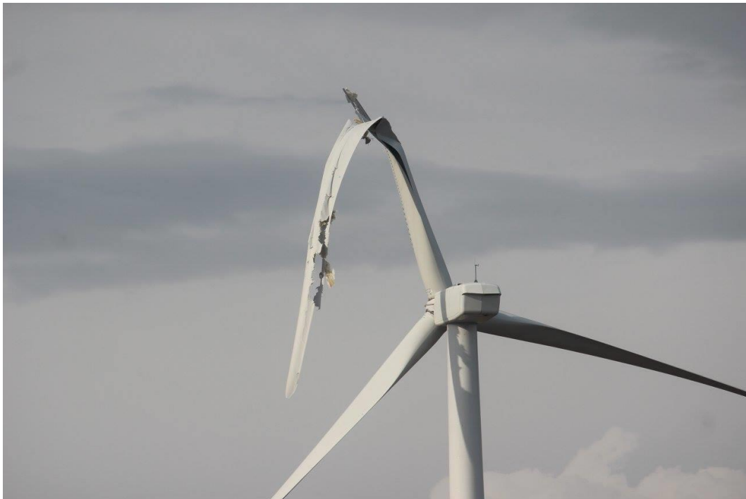
Figure 1.2: Example of blade's damage due to wind gusts.
