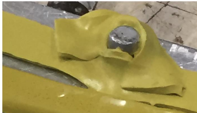
Figure 5.16 Sealant tape application
