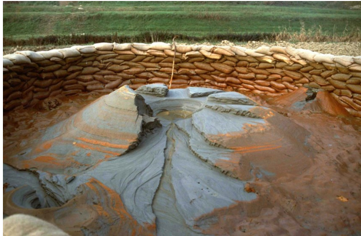
Figure 1.11: Piping phenomenon below the levee of the Po River.
