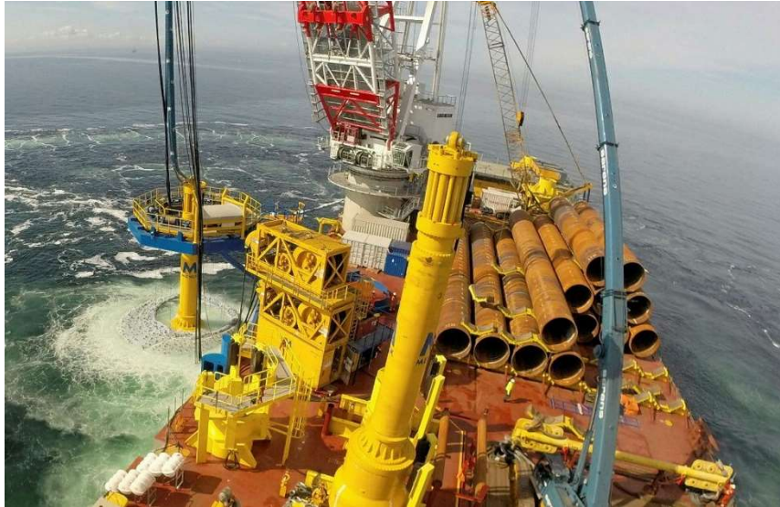
Figure 46: Offshore pile driving operation
