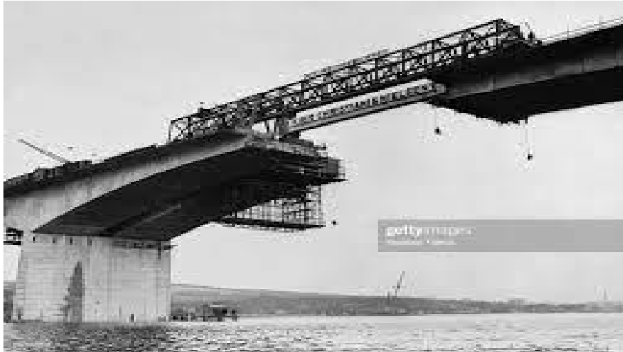
Figure 1.4. Medway viaduct under construction with the balanced cantilever method (Menn, 1986)
