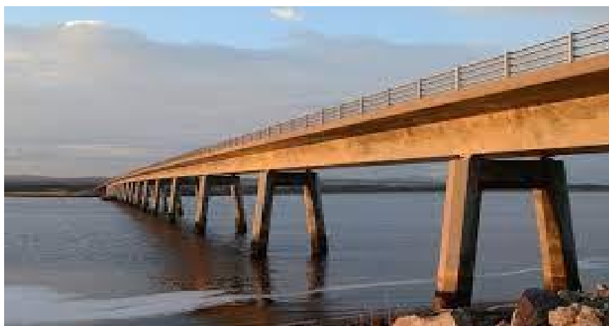
Figure 1.5. The bridge of Dornoch firth crossing, Scotland. (Maxwell, 2006)
