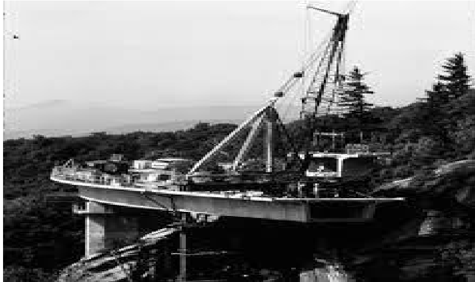
Figure 1.3. Linn cove viaduct under construction with precast segmental deck (Menn, 1986)
