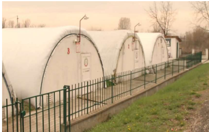
Figure 24, Part of Ekofungi facilities (production tunnels), source: courtesy of the founder
