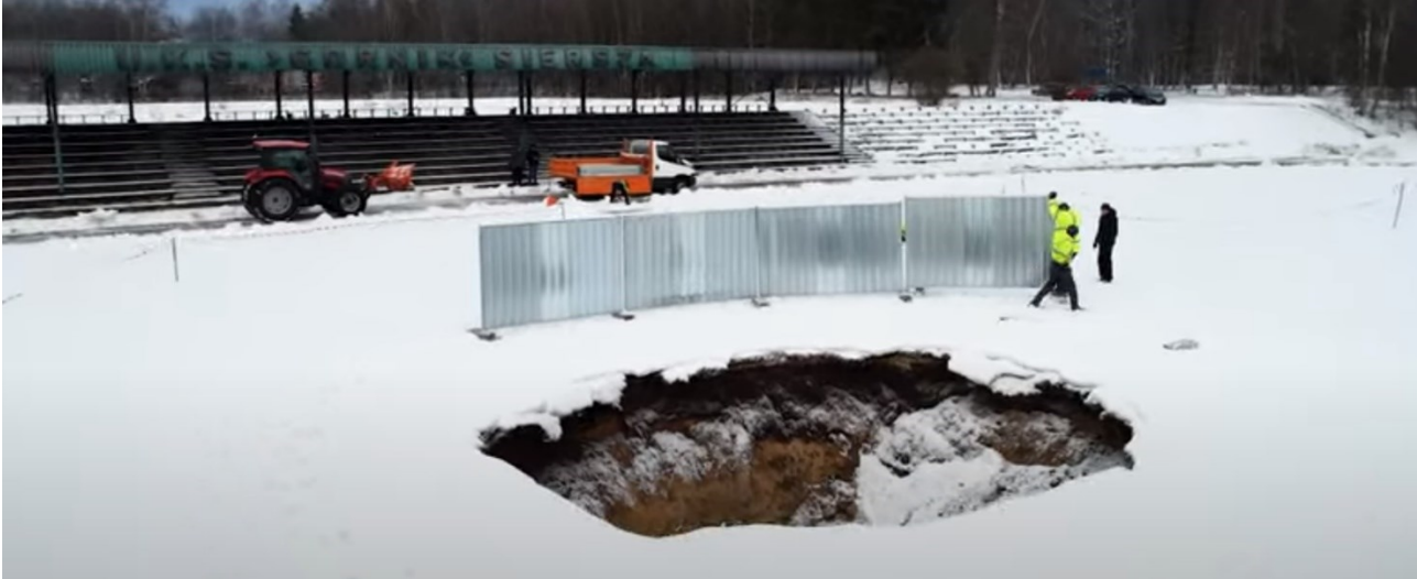
Figure 2.16 Sinkhole appeared in a football field, Trzebinia. Source: (Sinkholes in Trzebinia. There Are Test Results of the SRK Recovery Plan and Plan)
