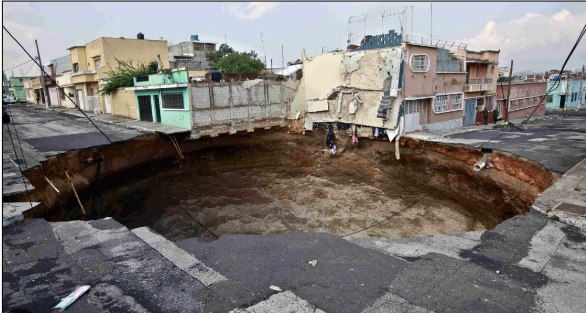
Figure 2.14 Lateral view of sinkhole in zone 2. Source: (Guatemala City Hit by Second Sinkhole | New Civil Engineer)
