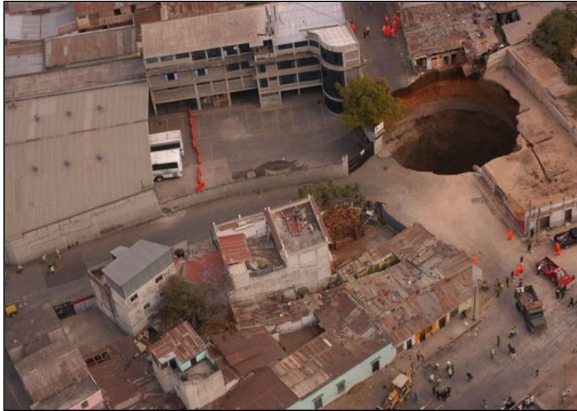
Figure 2.13 Sinkhole that occurred in zone 6. Source: (Hermosilla, 2012)
