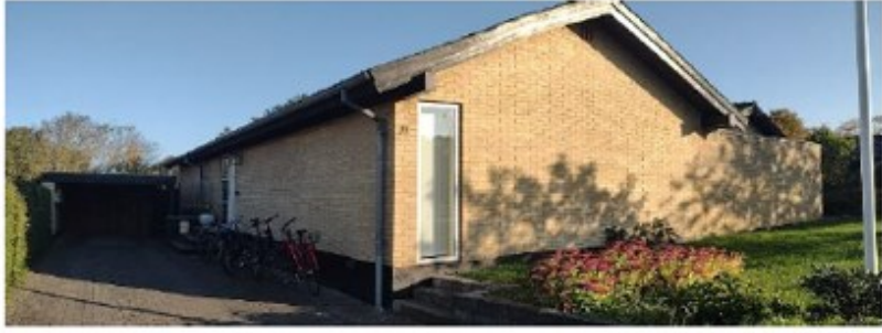
Figure 2-2: Picture of the single-family house (North-west) [9].
