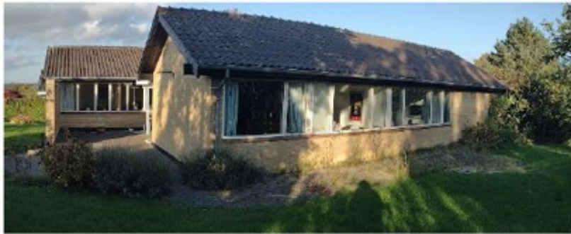
Figure 2-3: Picture of the single-family house (South) [9].
