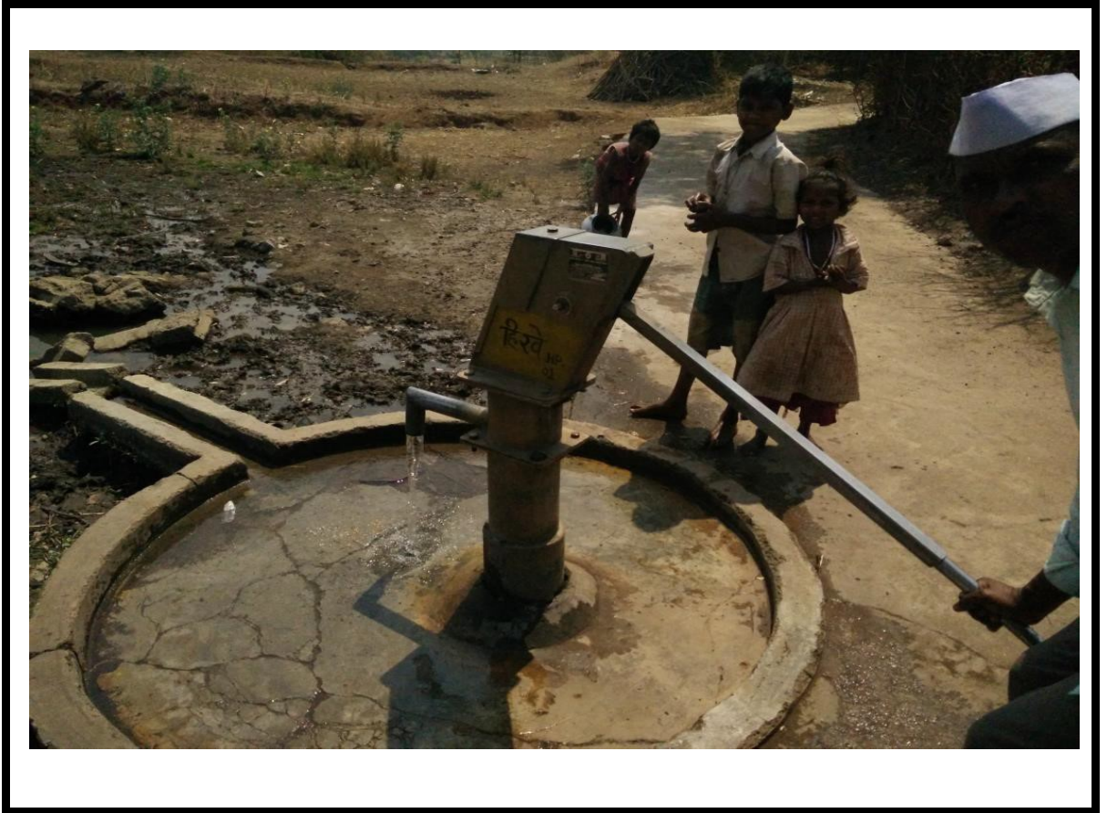
Figure (2.3): Some pumping methods in Sudan [3]
