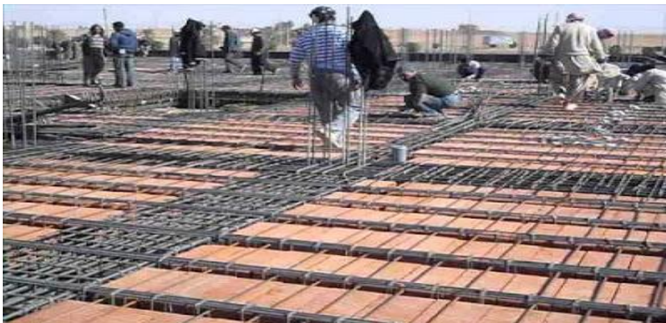
Figure1.6. Hardy floor construction (www.civilread.cm, 2021)
