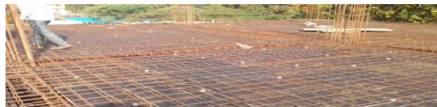
Figure1.3. Two way floor construction (www.civilread.cm, 2021)
