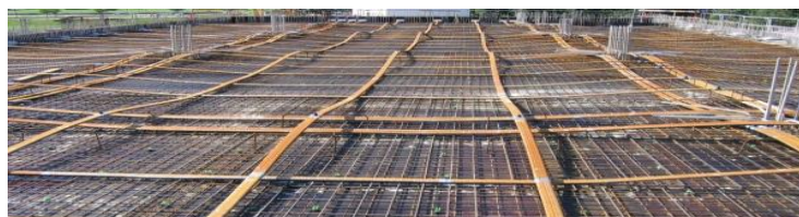
Figure 1.9. Post-tensioning floor construction (www.civilread.cm, 2021)
