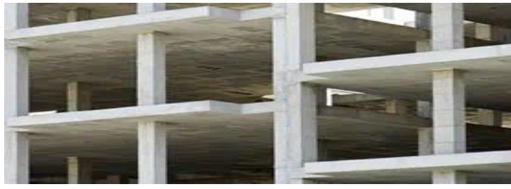
Figure 1.2. Flat floor construction (www.civilread.cm, 2021)
