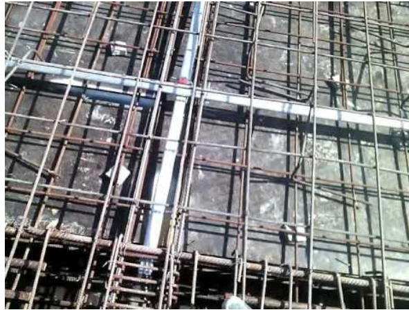
Figure1.8. Pre-tensioned floor construction (www.civilread.cm, 2021)
