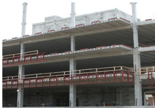
Figure1.7. Hollow core floor construction ( www.civilread.cm , 2021)
