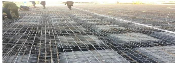
Figure1.5. Waffle floor construction (www.civilread.cm, 2021)
