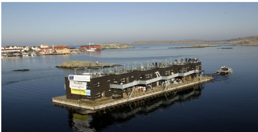
Figure 13 Salt & Sill Hotel in Sweden
