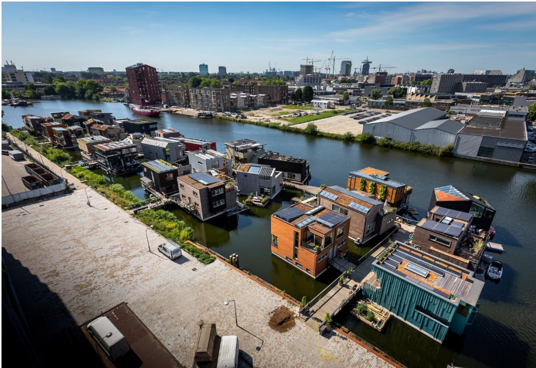
Figure 10 Floating Home Development in Amsterdam
