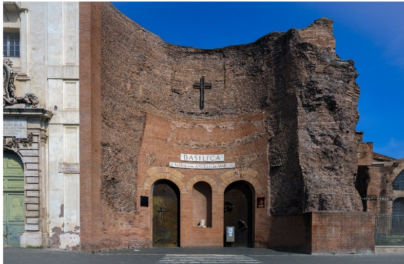
Figure 6 The church facade: an apse in the wall of the caldarium of the Baths of Diocletian
