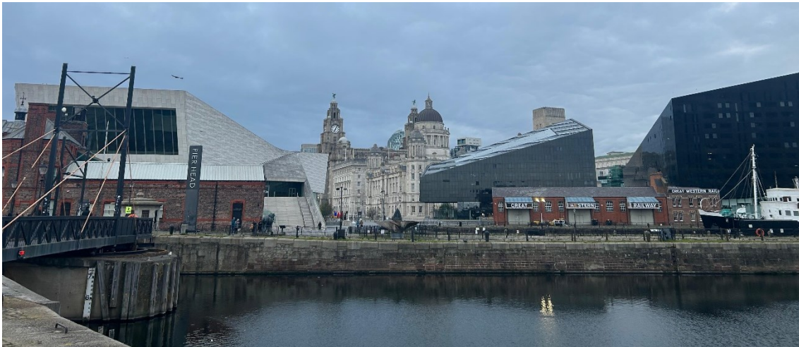
Figure 5 Pier Head view from Canning Dock (from left to right: Museum of Liverpool, the Three Graces, RIBA North). The blend of modern, 20 th -century and historic industrial architectural style create a unique atmosphere.
