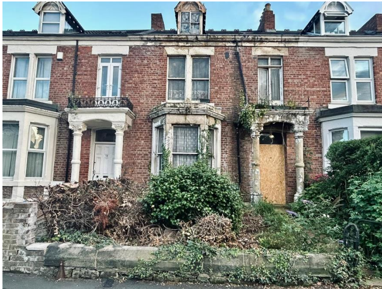
Figure 24 Private property in Heaton (Chiara Zannelli 2024)
