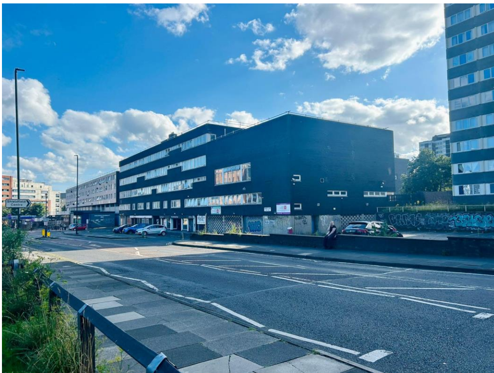
Figure 27 The Shieldfield Centre, the frontier of Heaton and Shieldfield (Chiara Zannelli 2024)
