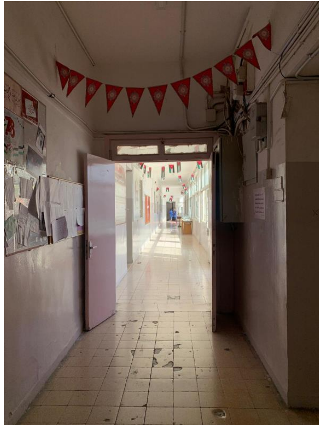
Figures 16, Corridors at the first and second floor of the Al-Hussein School for Girls in Jabal Hussein (picture of the author – 12/09/2024)
