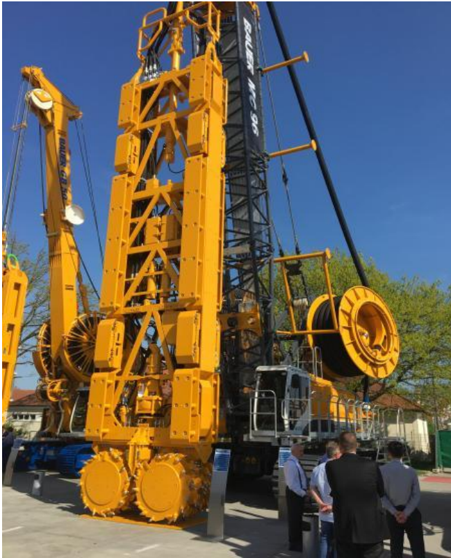
APPENDIX 8: Hydraulic drilling machine of diaphragm wall
