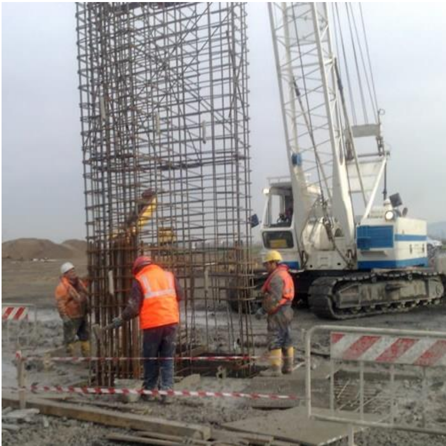
APPENDIX 9: Reinforcement cage of a panel of diaphragm wall
