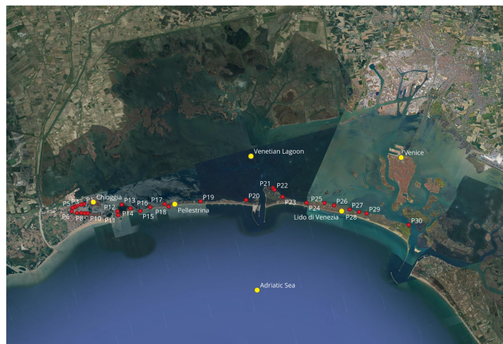
Figure 3. The locations of the 30 seawall's samples taken from Lusenizio, Pellestrina and Lido.
