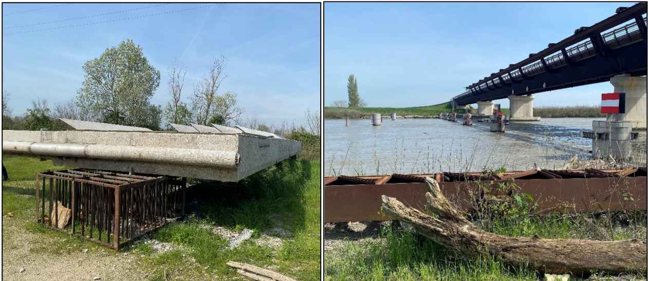
Figure 34 - Left: mobile salt barrier removed for maintenance; Right view of mobile salt barrier in the Po River
