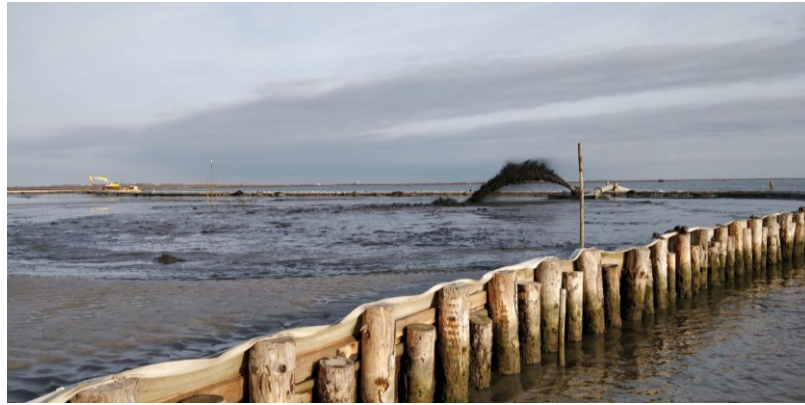
Figure 2.3. Disposal of dredged soil and water mixture at Le Sorelle-B via pipeline and hydraulic pumping.
