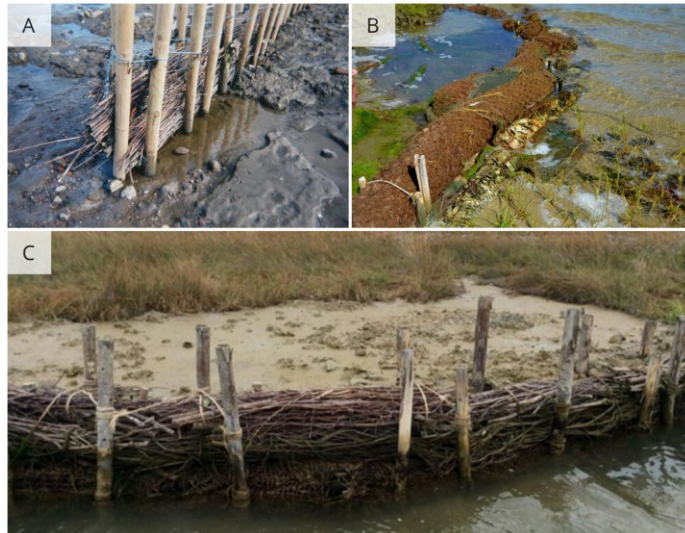
Figure 2.4. Salt marsh edges protection structures and sediments trap.
