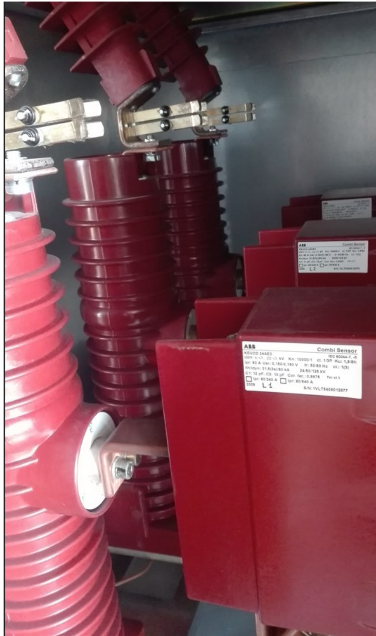
Fig.13 ABB COMBI KEVCD24AE3 photographic survey
