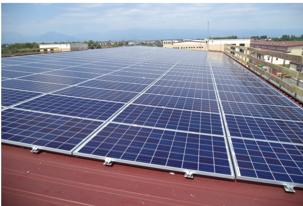
Fig.8 PV photographic survey
