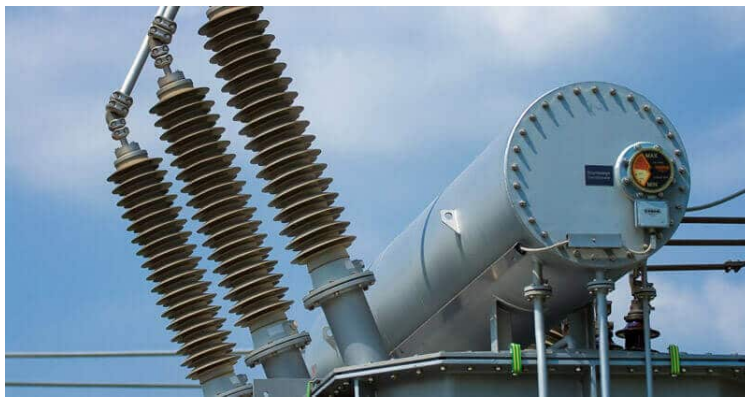
Figure 1.9: Transformer Bushings
