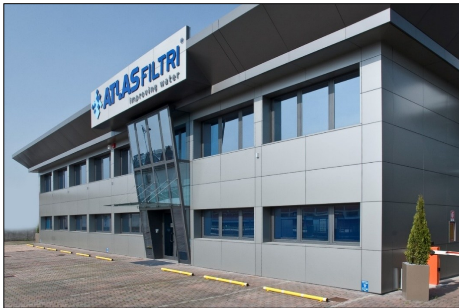
Fig. 0.1 Operational headquarters of Atlas Filtri company
