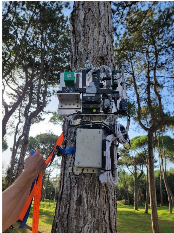
Figure 3. The sensor array installed in T_1 at H_{1/7} .
