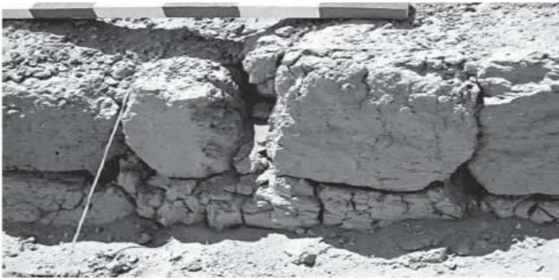
Figure 5. Sedimentary clay blocks of Ánimas commonly used for construction (Bachir Bacha & Llanos, 2013).
