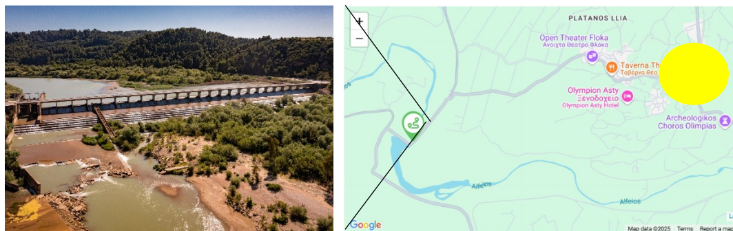
Figure 17: Alphiose Dam, Greece, source: Axis of katakolo, ancient Olympia R.W.G.
