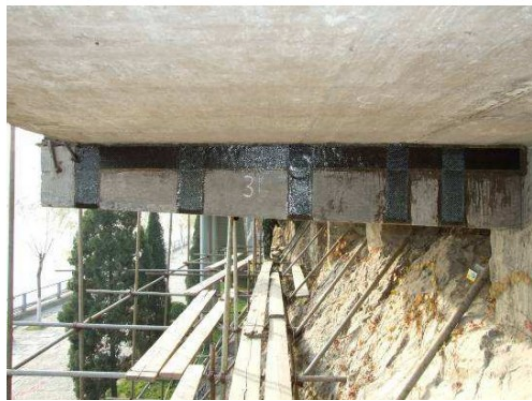
Figure 24: CFRP strips wrapped on the beam, Longmen site
