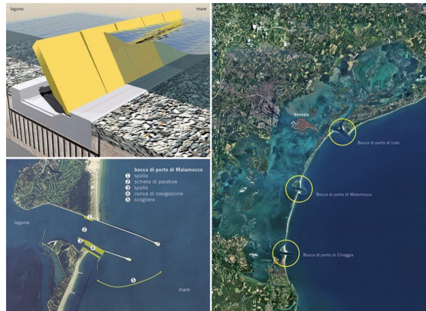
Figure 31: Mose flood barrier/ https://www.dutchwatersector.com/news/strukton-awarded-contract-to-immersed-caissons-for-venice-storm-surge-barrier
