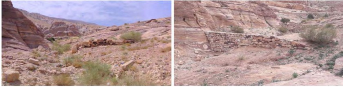
Figure 20: Reconstruction of dam (left : before)(right :after)
