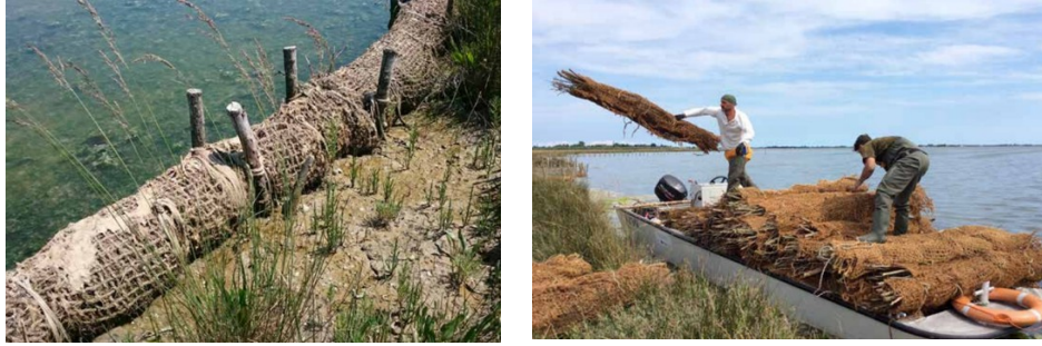
Figure 32: Soil-bioengineering techniques against erosion, (source: brief of LIFE VIMINE , Venice integrated management of intertidal environments)
