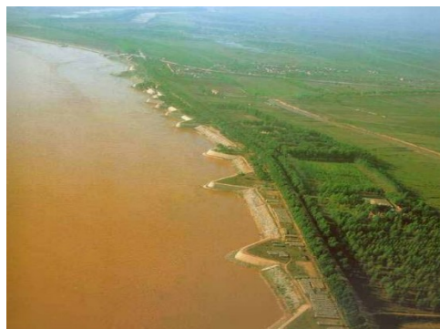
Figure 27: Levee protection works, stone masonry spur dike
