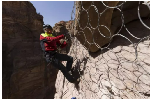
Figure 21: Stabilization of rock in Petra site by UNESCO
