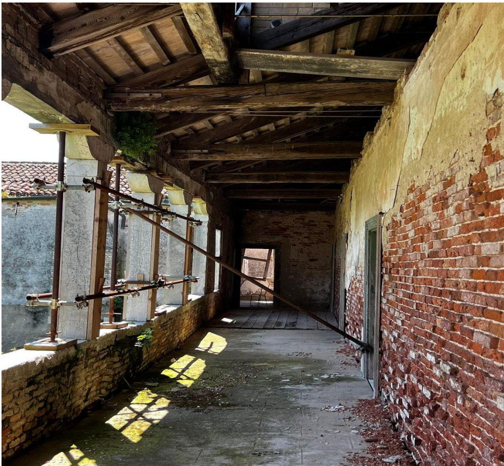
Figure 70. Covered passageway on the upper floor.
