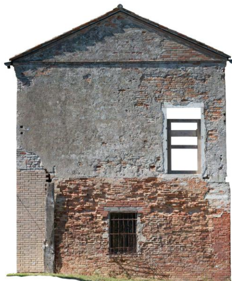
Figure 34. Second east (E2) exterior façade of the Generalato.
