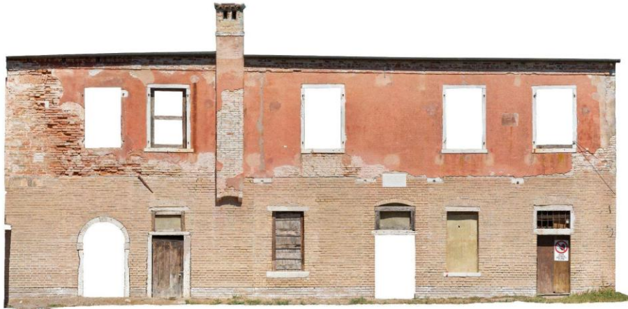
Figure 25. South (S) exterior façade of the Generalato.
