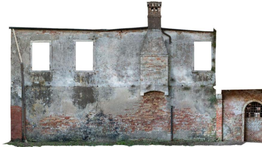
Figure 33. Second north (N2) exterior façade of the Generalato.
