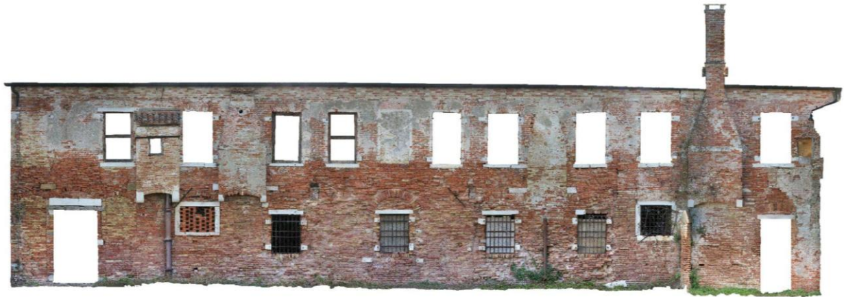
Figure 24. West (W) exterior façade of the Generalato.
