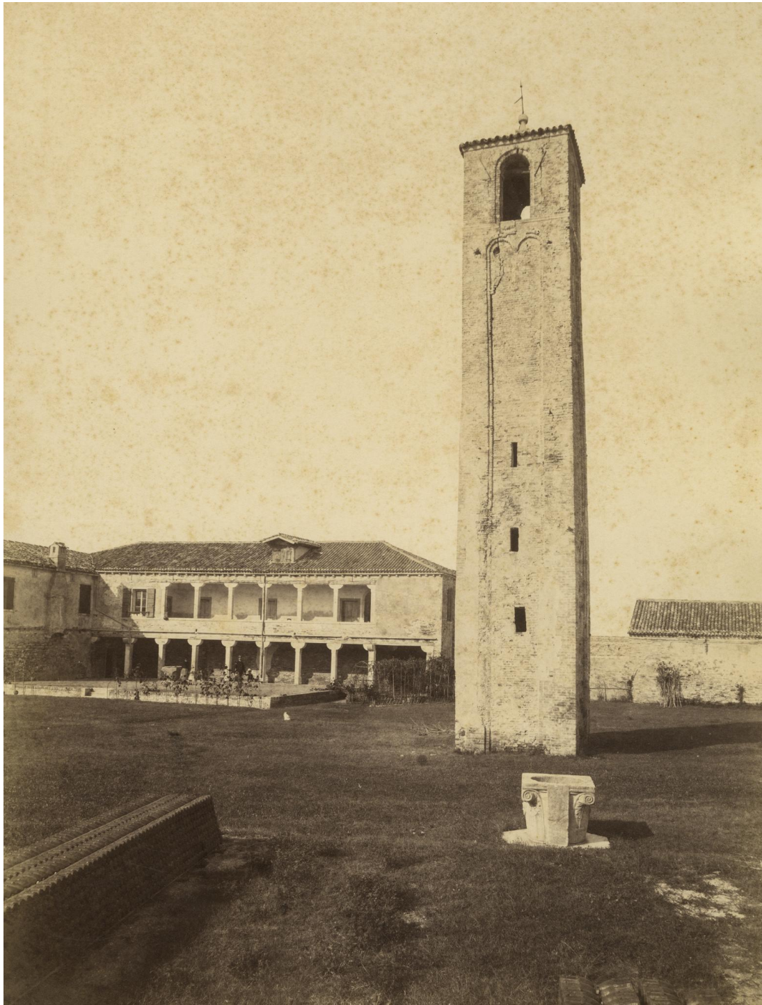
Figure 18. Picture of the bell tower and the Generalato in the late 19 th century, after the demolition of the church and half of the ancient monastery, taken in 1889 (Correr Museum, inv. MCV-CF001345).
