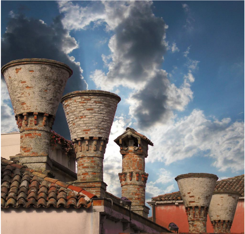
Figure 61. Traditional chimneys “a campana” in Venice.
