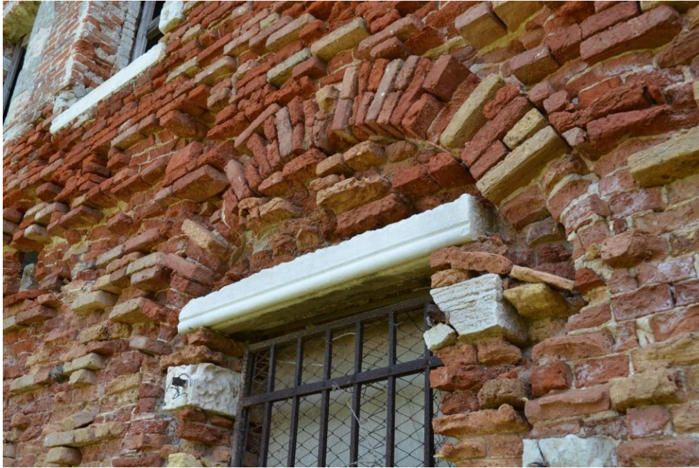
Figure 44. W façade of the Generalato, displaying detachment patterns analysed and identified by the “Material disintegration” category.
