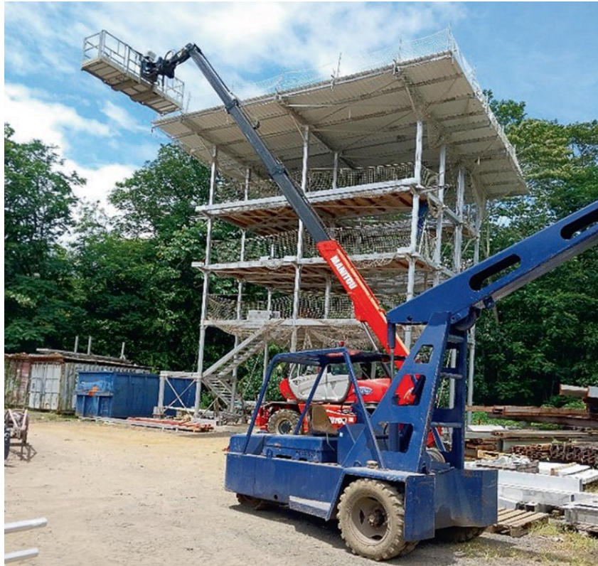
Figure 36: Construction of the aluminum tower (Source: VAOT association).
