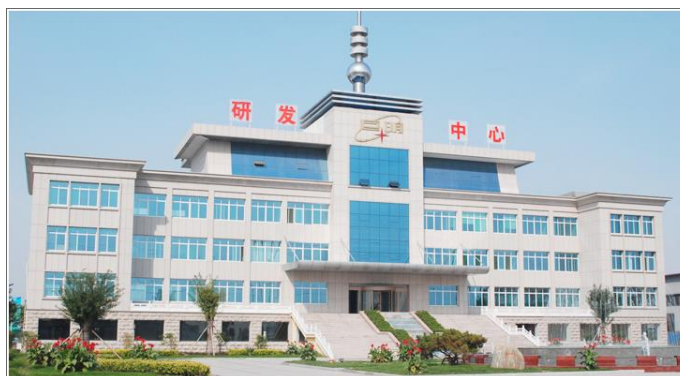
Figura 18-Headquarter di Shandong Juming Group a Zibo, China.
