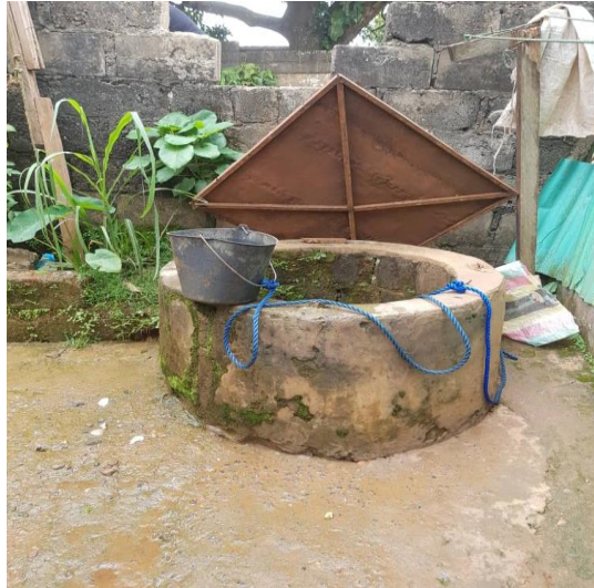
Figure 21 :Well1 situated in a family compound equipped with a metallic lid
