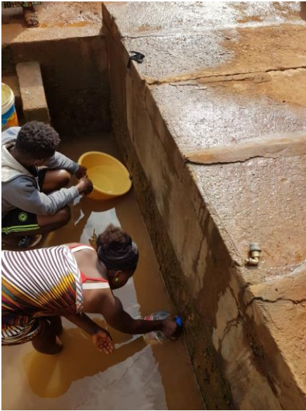
Figure 26: Collection of water from spring through the 2 piped outlets
