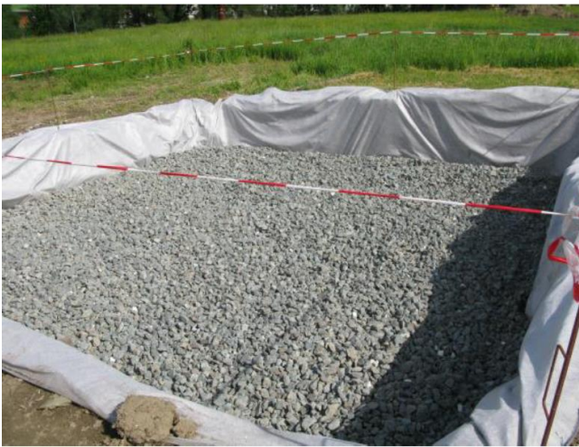
Figure 3.4 Photo of the biowindows' GDL (Hrad and Huber-Humer, 2015)
