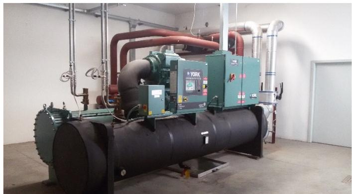
FIGURA 15 – MACCHINA FRIGORIFERA YORK DOTATA DI COMPRESSORE CENTRIFUGO
