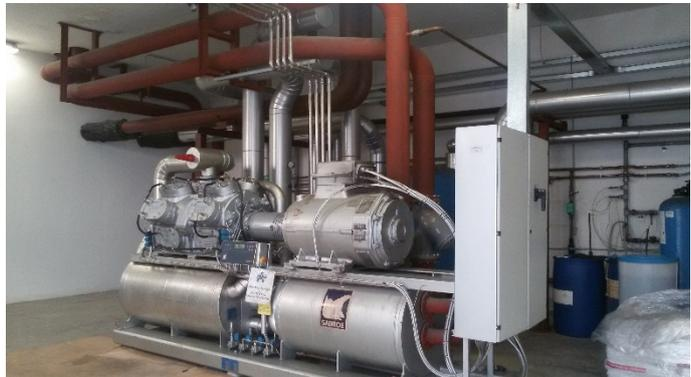
**FIGURA 16 – MACCHINA FRIGORIFERA SABROE DOTATA DI COMPRESSORE ALTERNATIVO**
