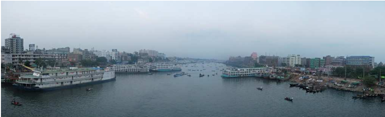
Photograph 3.1: View of Buriganga River from the bridge-1 in Dhaka. Picture Credit-Rangan Datta.
