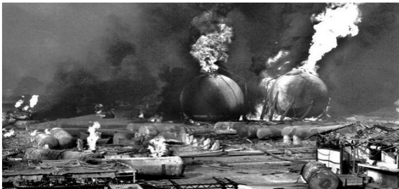
Figure 1.4: San Juanico site after tanks explosion. A part of the LPG still burns.
