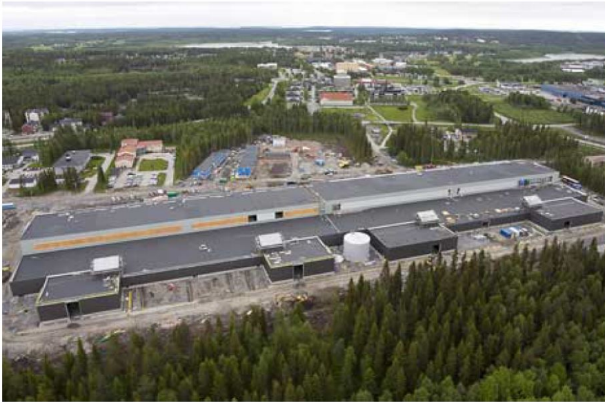
Figure 1.2: Aerial view of the Facebook data center in Luleå, Sweden.
