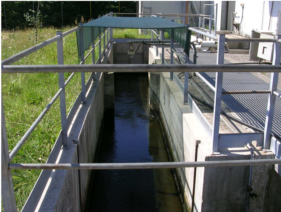
Figure 5.1 – San Donà di Piave WWTP final discharge channel after the contact tank
