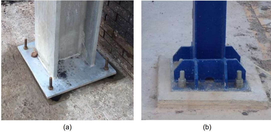
Figure 1.4. Conventional exposed cross-section column bases: (a) unstiffened H-section column base; (b) stiffened H-column base (Kamperidis, 2016)
