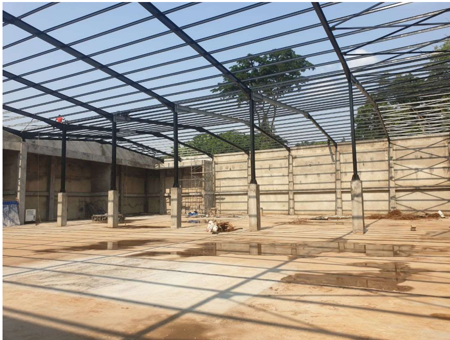
Figure 3.3. Ware house for stockage at Odza
