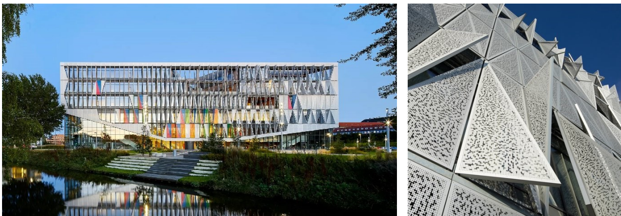
Figura 2.1.1: Involucro adattivo del SDU Campus Kolding, Henning Larsen Architects, Danimarca, 2014.
