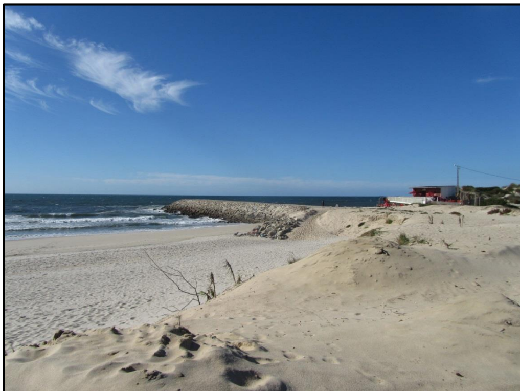
Figure 5.5. Vagueira South groin seen from land. Site visit on October 2012.
