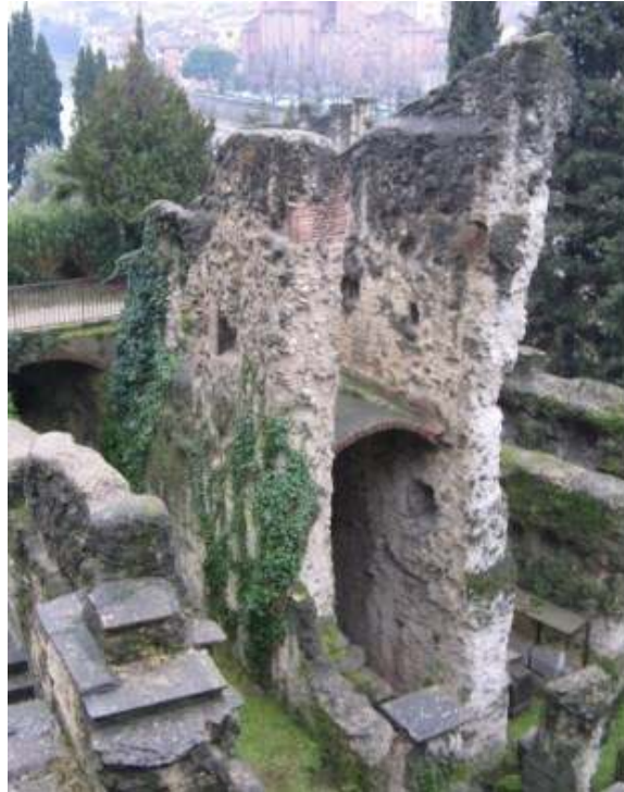
Figure 1.4c - Western radial walls of the cavea
