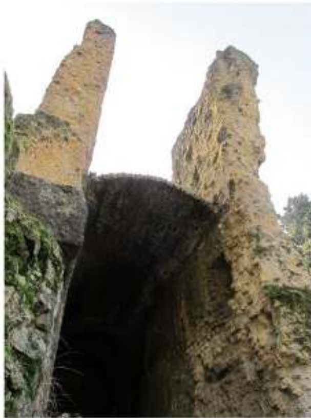
Figure 1.4b - Western radial wall of the cavea
