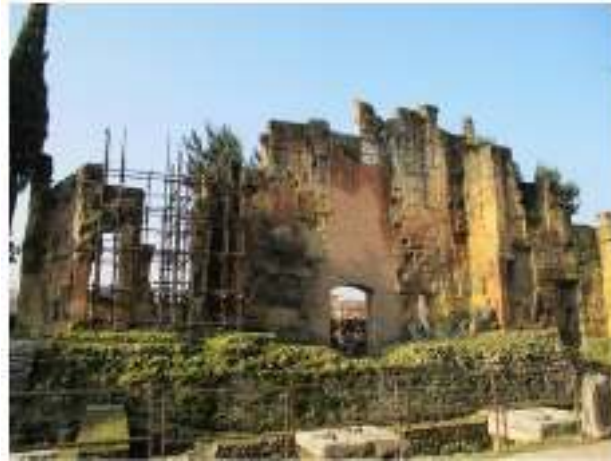
Figure 1.4a - Internal view of the stage building
