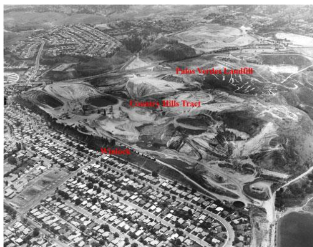
1963 Disposal Gardens (now Country Hills tract) and Palos Verdes Landfill
