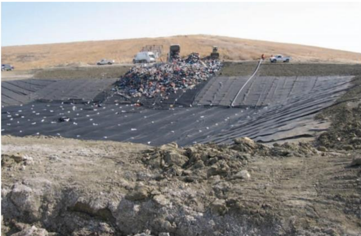
Figure 1.13. Filling operation of Calgary Biocell.
