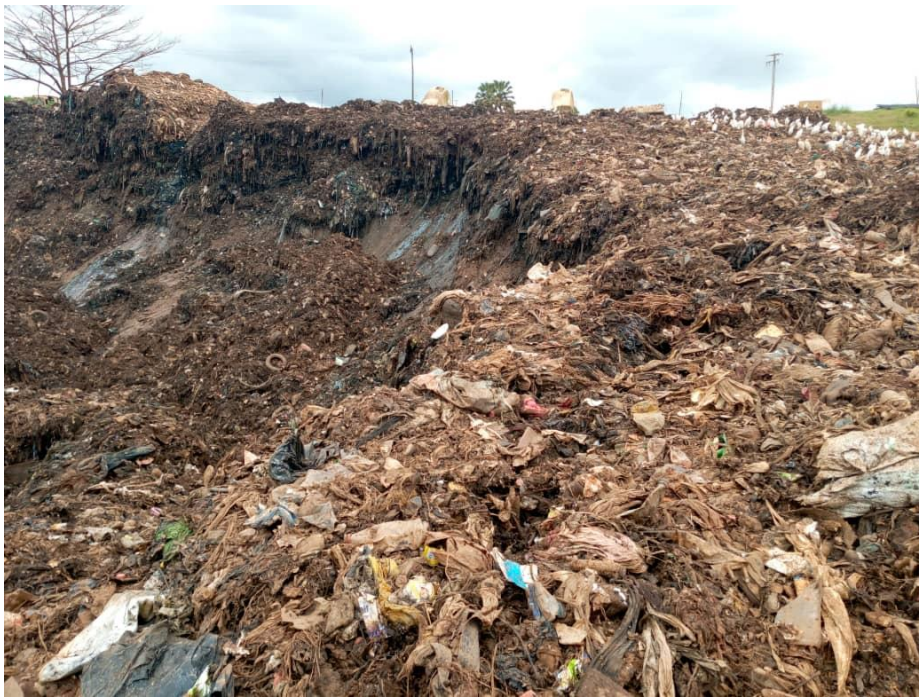
Figure 3.7. Presentation of the first landslide in the Nkolfoulou landfill (July, 2019).
