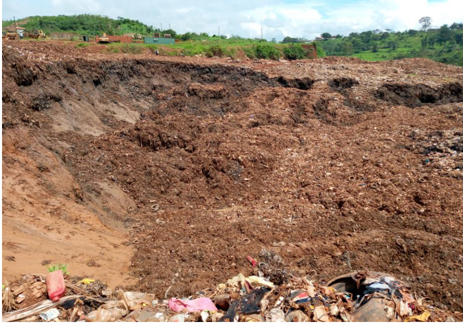
Annex IV. Presentation of the second landslide in the Nkolfoulou landfill (October, 2019).
