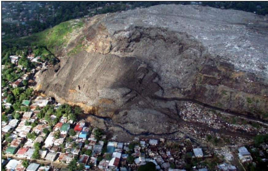
Figure 1.12. Picture of landslide landfill Payatas, Quezon City, Metro Manila, Philippines (Jafari, Prof. Tim Stark and Prof. Scott Merry, 2000).
