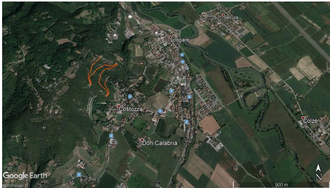
Fig. 7: view of Santa Tecla section. Image from Google Earth.
