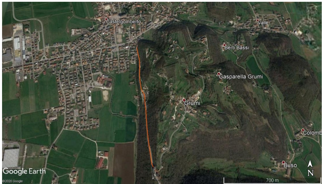
Fig. 5: View of the Castelvomberto section. Image from Google Earth
