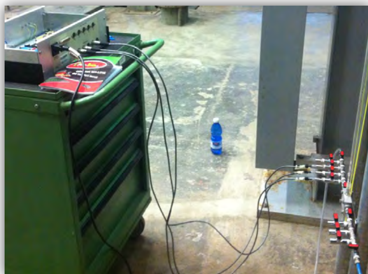
Figure 3.7: Particular of the connection between the column, the sensors and the conditioning unit;
