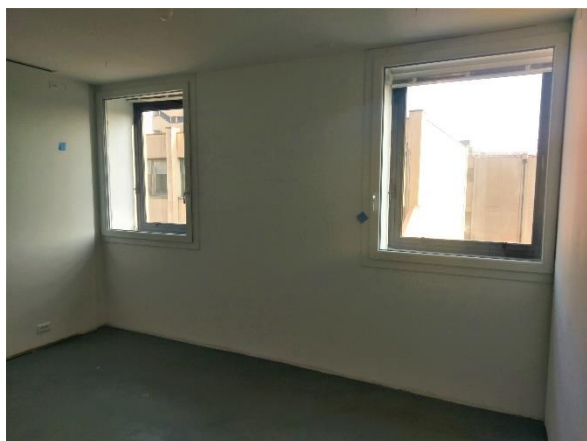
a) Details of east wall and windows.
