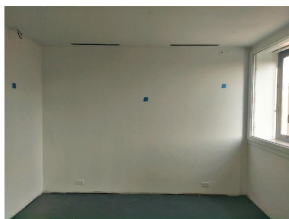
d) Details of north wall and delivery vents on the ceiling.
