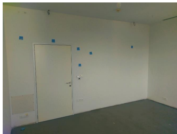
b) Details of west wall and door.
