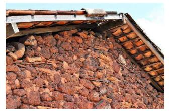
Figure 79 Wall made of *pedra e barro* and without the wall plaster in a house of Ouro Preto. Photo by Elio Moroni Filho. Source: Moroni Filho [2020].<sup>296</sup>
