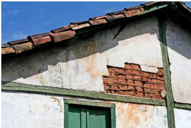
Figure 85 Pau-a-pique used to seal the wood structure of a house in Ouro Preto. Source: Machado [2009]<sup>303</sup>.
