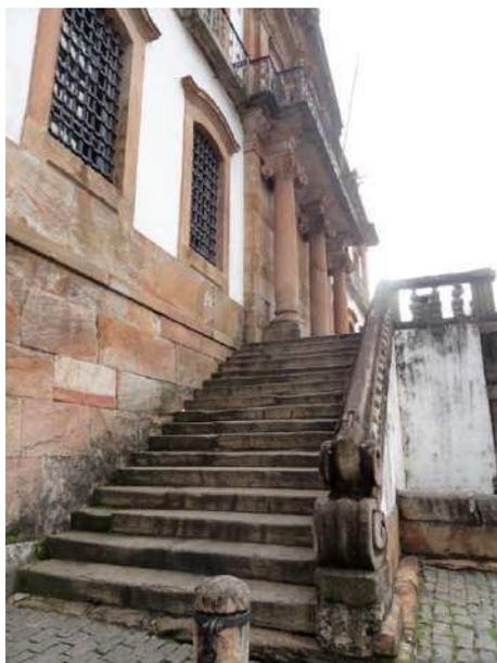
Figure 81 *Pedra e cal* masonry, used in the *Museu da Inconfidência*. We can as well see stones used in other elements, like the stairs, columns, lintels, sills, etc. Source: Gagliardi, 2019.<sup>298</sup>
