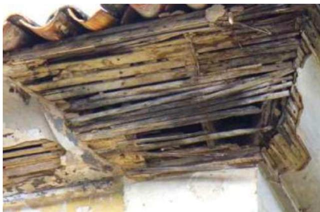
Figure 86 Use of the estoque in a cymatium in Ouro Preto. Source: Martins [2010]<sup>304</sup>.
