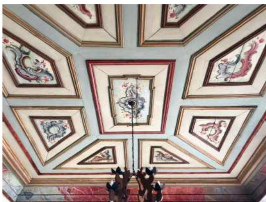
Figure 88 Framed panel ceiling found in Casa dos Contos. Source: Viajento [2018]<sup>307</sup>.
