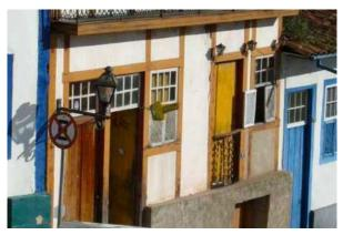
Figure 89 Example of the openings of a house, with their painted beams, sills, and jambs. It is possible to observe the elongated beans and jambs, and the use of the same bean for different openings. Source: Martins [2010]<sup>308</sup>.
