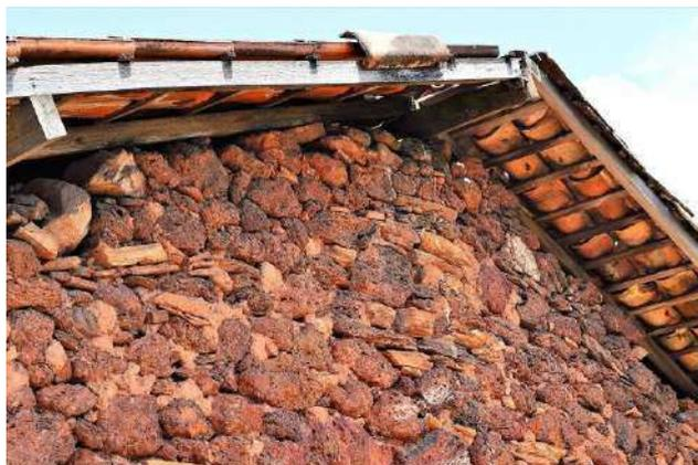
Figure 79 Wall made of *pedra e barro* and without the wall plaster in a house of Ouro Preto. Photo by Elio Moroni Filho.
