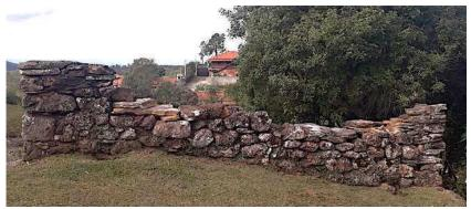
Figure 78 Wall made of *pedra seca* (dry-stone masonry) in Ouro Preto. Photo: author, 2018. Another type of stone masonry is the *pedra e barro* (stone and mud) (**figure 79**), in which is employed mud as mortar and the stones can be natural or worked to have a better finish.
